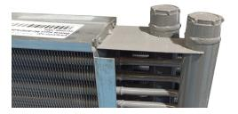
If a water leak has been detected in the battery, possible corrosion problems in both the battery and the curtain components should be checked.
