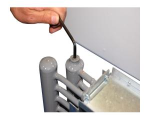
To remove the coil, unscrew the fixing screws as shown on the next page:
