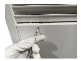
2. Remove the two safety screw from the service door.
