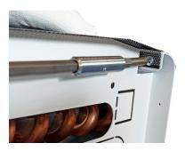
4. Unscrew the screws that hold the water coil.
