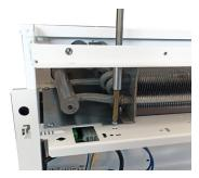
5. Drain the water battery with the drain plug of the main collector as shown in the photograph and disconnect the battery from the installation.
